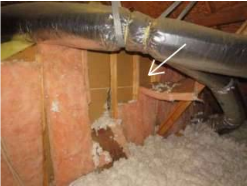
Photo 26-4 Insulation fallen
