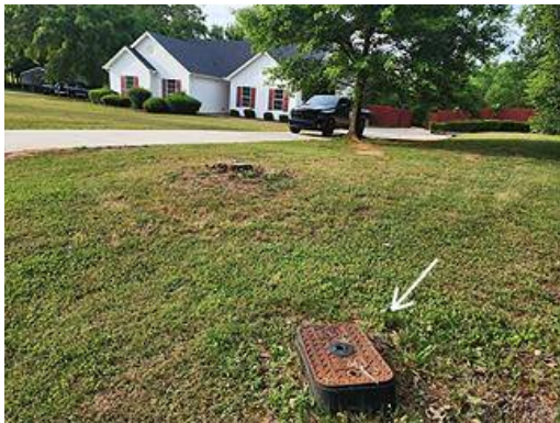
Photo 27-1 Front yard shut off location
