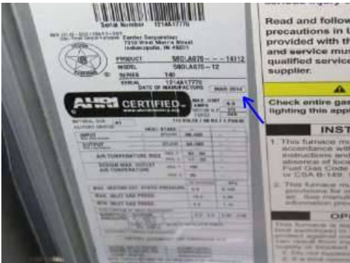
Photo 18-4 Manufactured 2014 Filter behind grill in hall, and at air handler base
