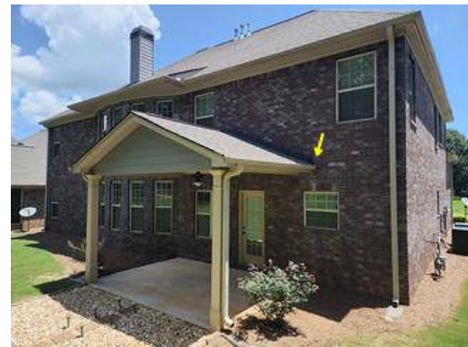
Photo 8-1 Both sides of patio cover
