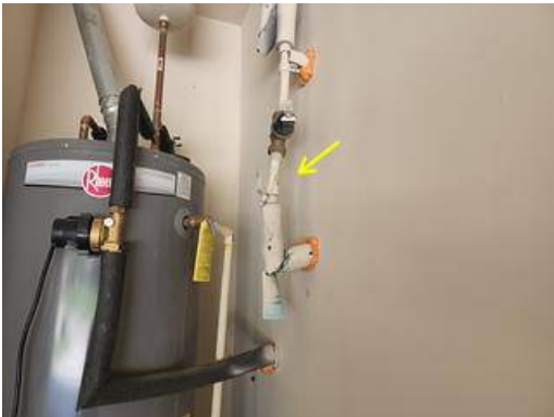
Photo 44-2 Garage shut off location
