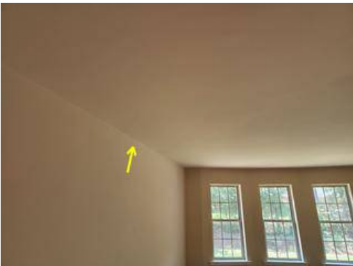
Photo 38-2 Living area ceiling
