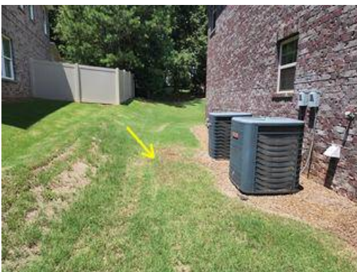
Photo 2-1 Left side of home
