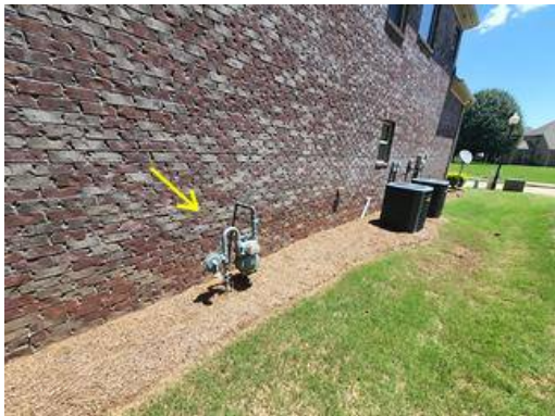
Photo 45-1 Left side of home
