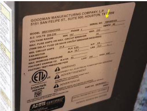
Photo 29-4 Manufactured 2018 3.5-ton unit
